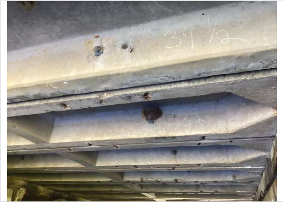
Bottom deck span 1
