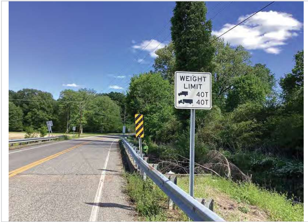
Weight limit sign Opposite Direction of Route
