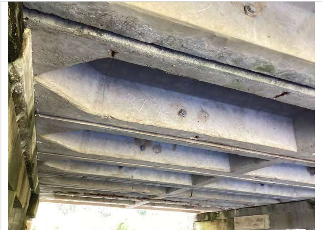
Bottom deck span 2
