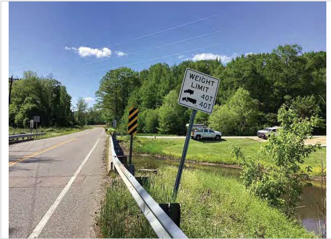
Weight limit sign Direction of Route
